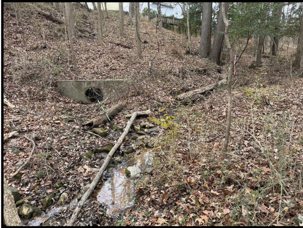
PHOTO 9: Storm drain outfall on right (south) bank at lower end of site.
