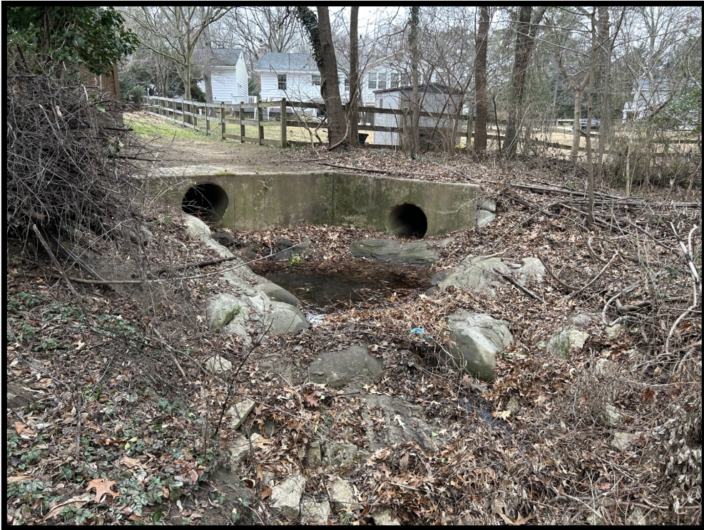
PHOTO 1: Outfalls at upstream end of project.
